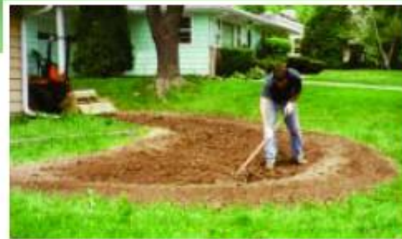
On a gentle slope, soil from digging out the garden can be used to create the berm. This rain garden is 4 inches deep.
