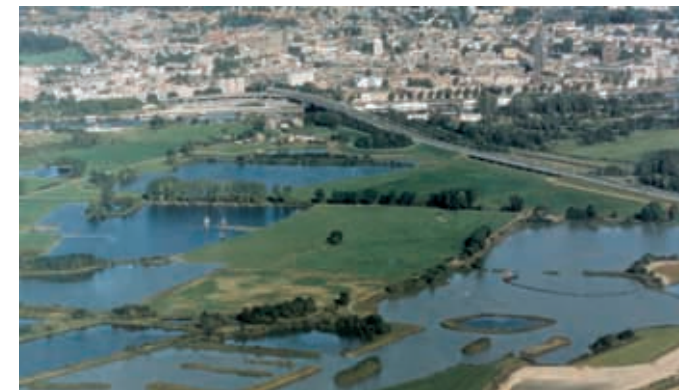
(6) The urban greenstructure and the main ecological structure meet and form one system, Arnhem and the river Rhine
