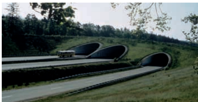
(5) Green corridors can cross traffic flows with special so called ecoducts
