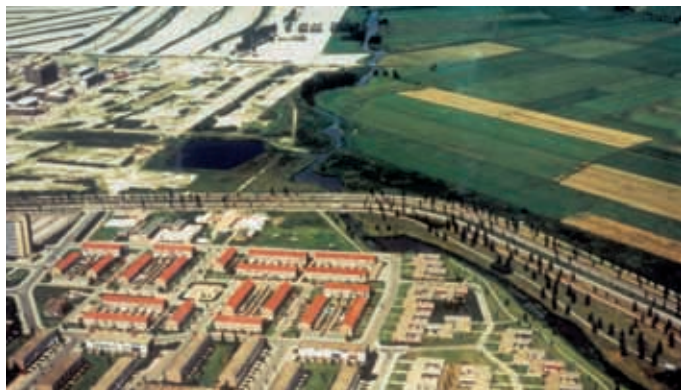
(3) An example of eco-inclusive planning during construction; Aa-landen in Zwolle Netherlands
